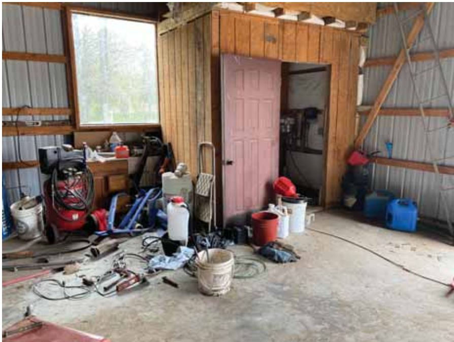
Photo 8: View of the sink and toilet area in the eastern interior of the pole barn building, which is suspected to discharge to a sanitary septic disposal system (REC-6).
