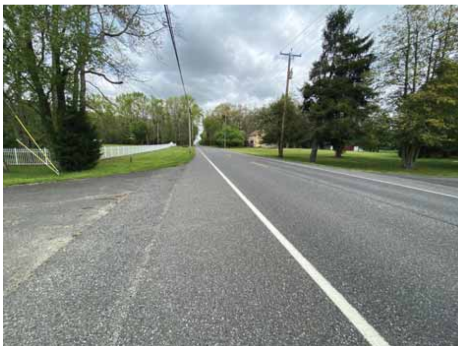
Photo 2: View looking northbound along Buck Road with the Site to the left.
