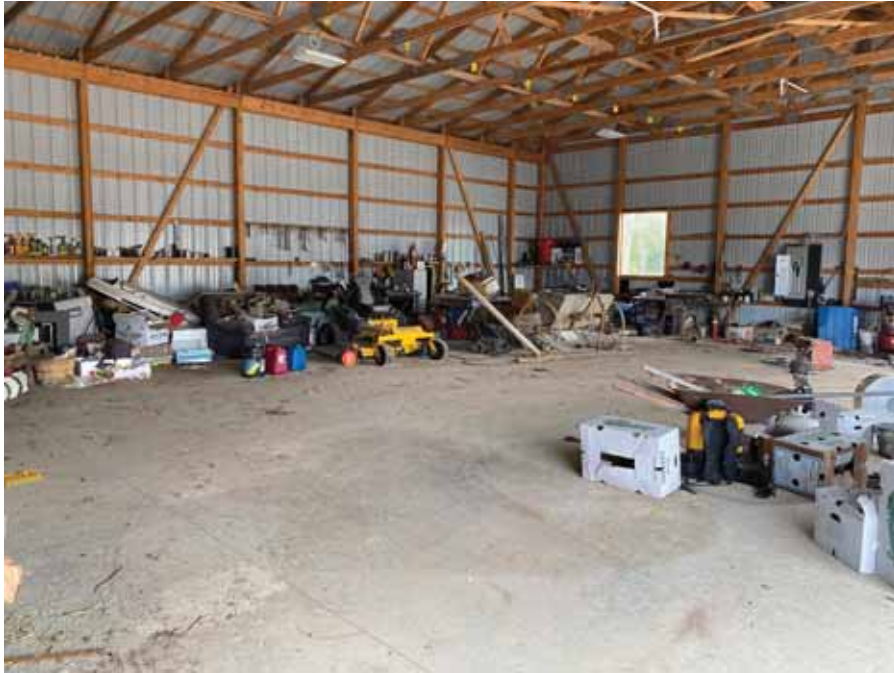
Photo 7: Representative view of the interior of the pole barn building onsite.
