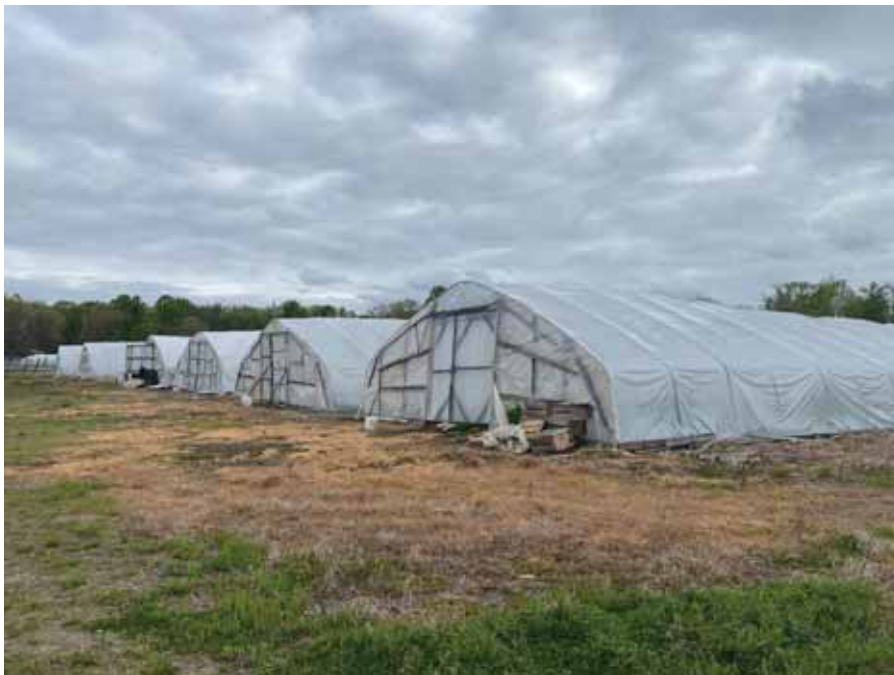
Photo 10: Representative view of the existing greenhouse buildings (REC-2) located in the eastern area of the Site.
