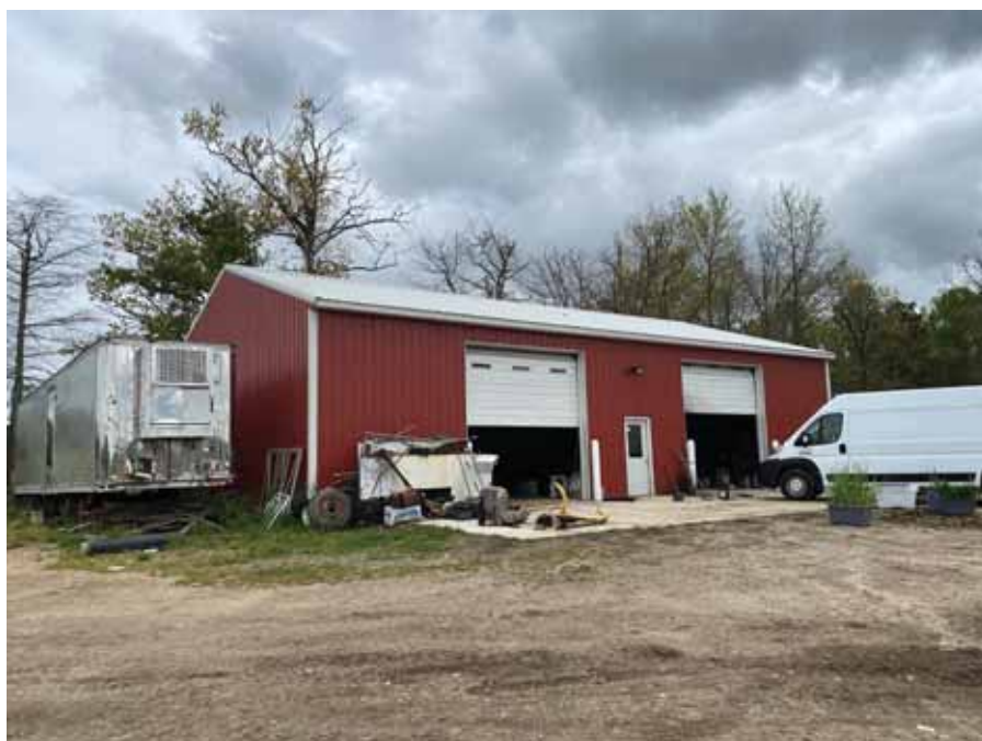
Photo 6: View of the pole barn building present in the northeastern area of the Site.
